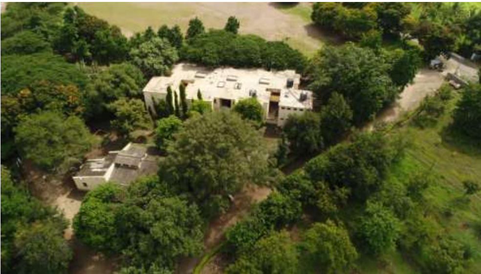
Aerial view of Boys Hostel
